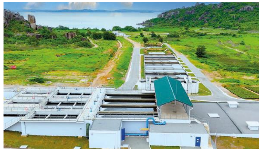
BUTIMBA DRINKING WATER STATION
